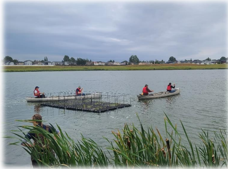
Figure 11: Installation of Floating Wetlands at Kensington 1 Pond
