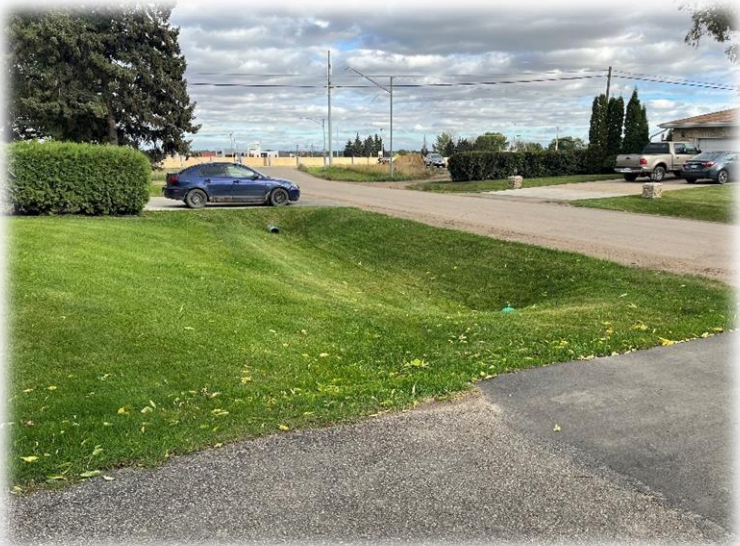
Figure 5: Completed Ditch Improvements in Montgomery Place
