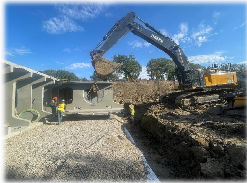
Figure 3: Installation of Underground Storage in Brevoort Park South
