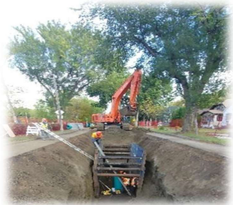
Figure 1.7 - Photo of Work in an Excavated Trench
