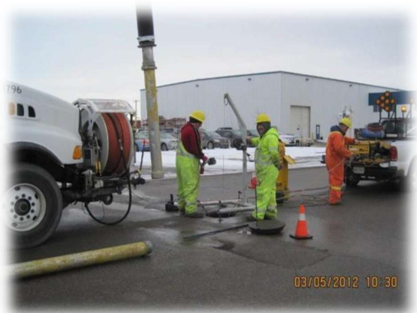
Figure 1.6 - Photo of Sewer inspection Activities
