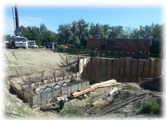
Figure 1.5 - Photo of Lift Station Infrastructure Construction
