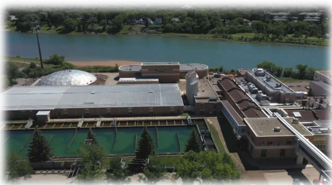
Figure 1.1 – Aerial Photo of the WTP
