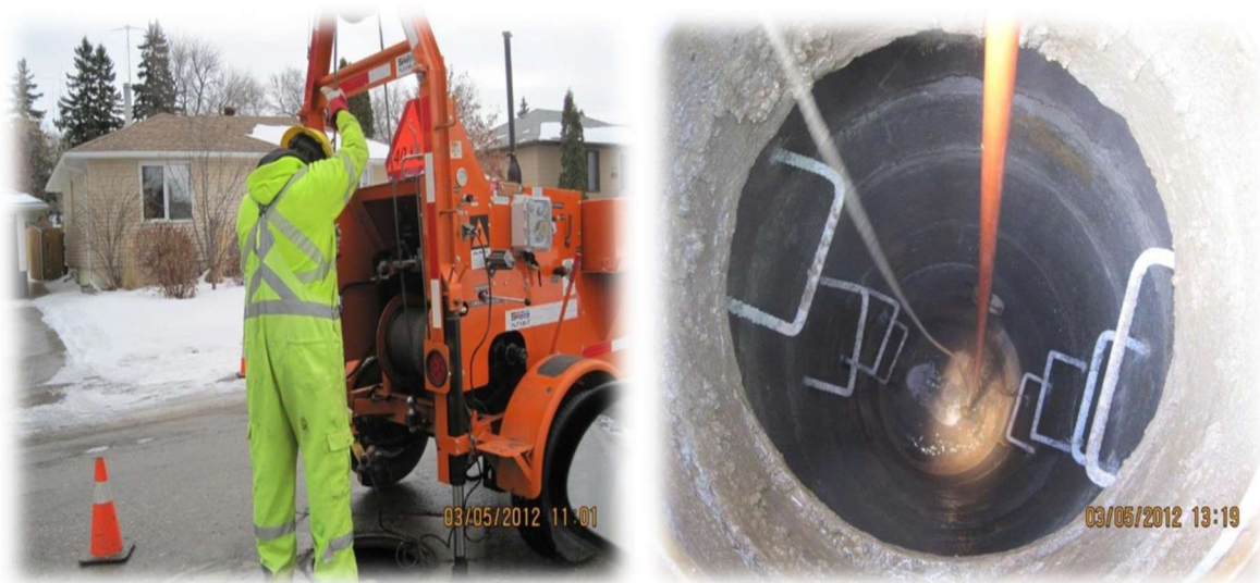
Figure 5.9 - Photos of Closed-Circuit Television Inspection Work
