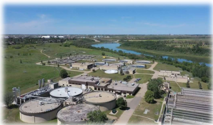
Figure 1.2 – Aerial Photo of the WWTP
