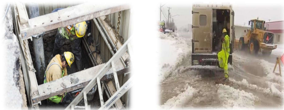
Figure 5.6 - Photos of Water Main Break Repair Work
