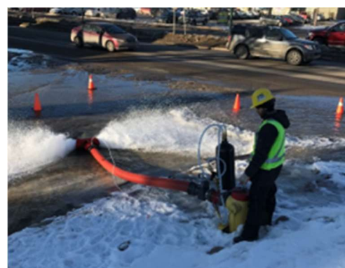
Figure 5.15 - Fire Flow Testing
