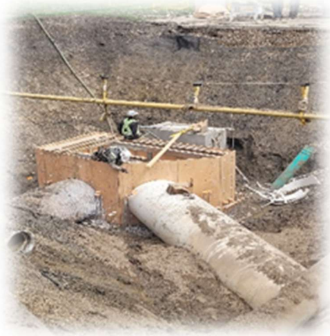
Figure 5.16 - Cumberland Storm Pond Chamber Installation
