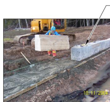
STEPED DISCHARGE WEIR WALL - FIRST STEP FOR LOW FLOW STORM EVENTS, SECOND STEP FOR HIGH FLOW STORM EVENTS THAT EXCEED THE CONTAINMENT CAPACITY OF THE WETLAND
